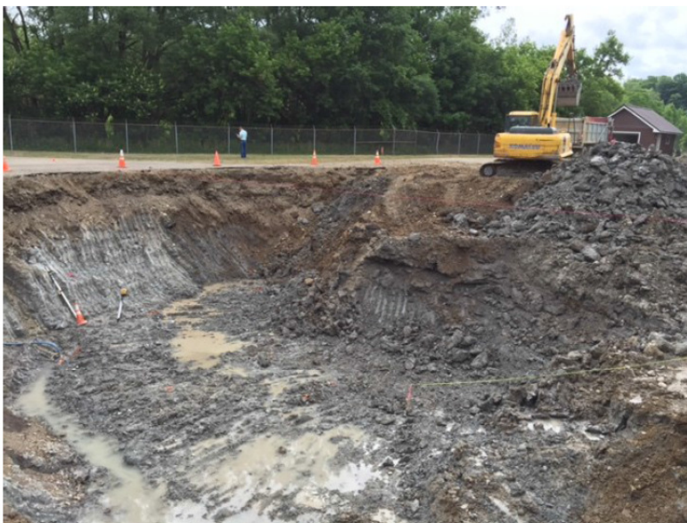
WWTF- Future Sludge Treatment Tank- excavation for tank construction 07/05/2016
